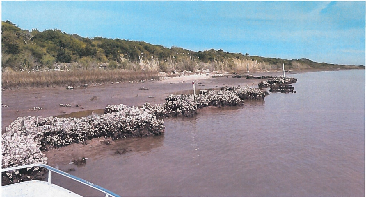
East end of the 1,000 feet of Reefblk installed in 2007 along Mad Island Marsh Preserve shore. This 1,000-feet of Reefblk will remain in place, unaltered. TNC observations are that marsh and oyster clumps have established behind the Reefblk. View towards the east from the GIWW. Photo by Freese and Nichols, Inc. on January 4, 2018 during very low tide.
