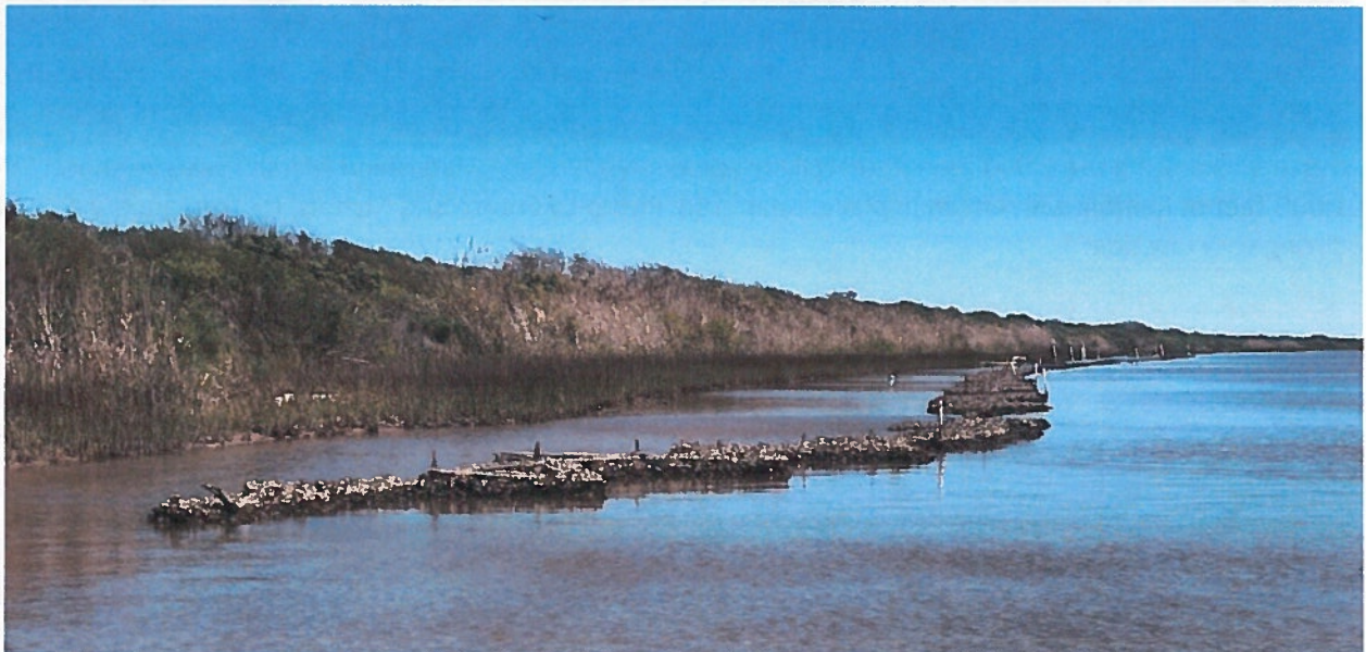
West end of the 1,000 feet of Reefblk installed in 2007 along Mad Island Marsh Preserve shore. This 1,000-feet of Reefblk will remain in place, unaltered. View towards the east. Photo by Freese and Nichols, Inc. on March 20, 2018.
