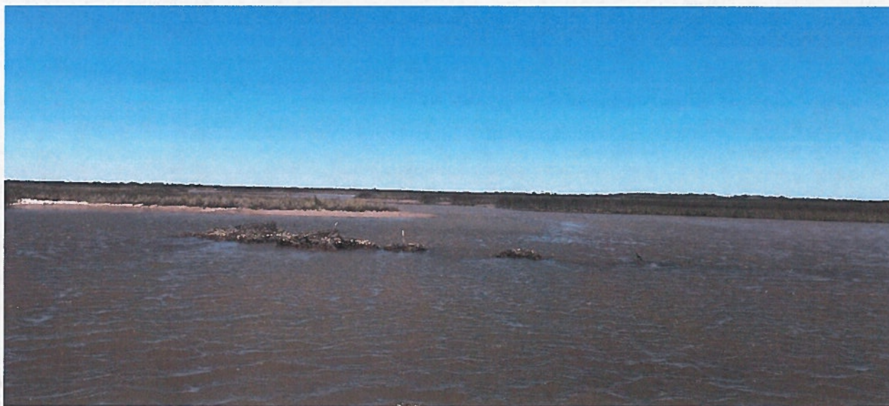
Damaged and fragmented Reefblk in front of the old mouth of Mad Island Bayou on Mad Island Marsh Preserve. View towards north from the GIWW. Photo by Freese and Nichols, Inc. on March 20, 2018.
